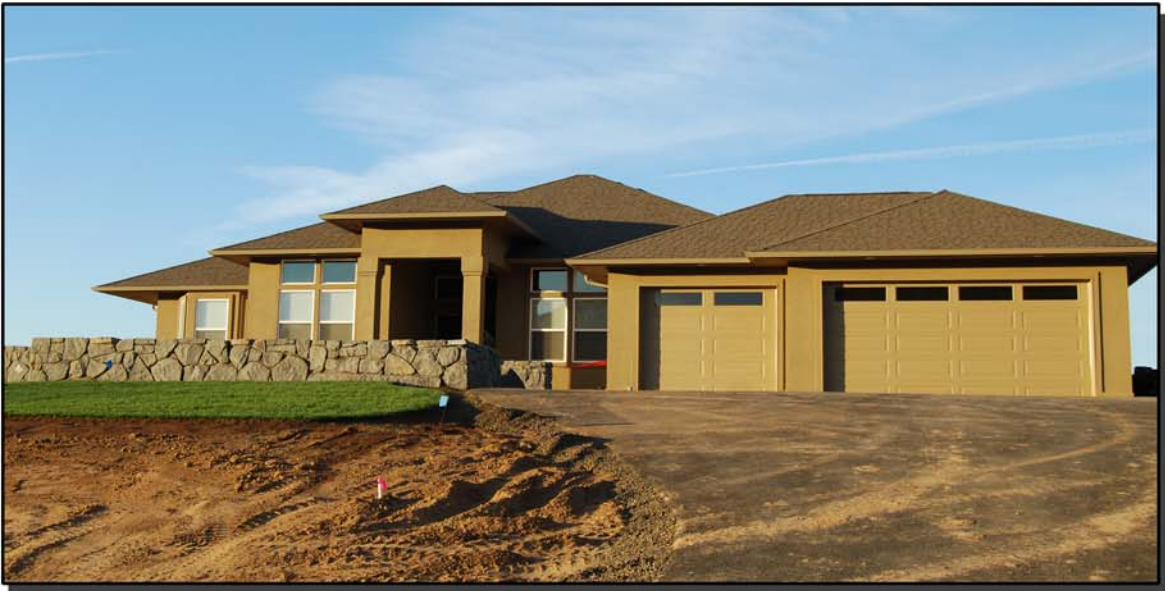
House #5 - New Creation Construction
